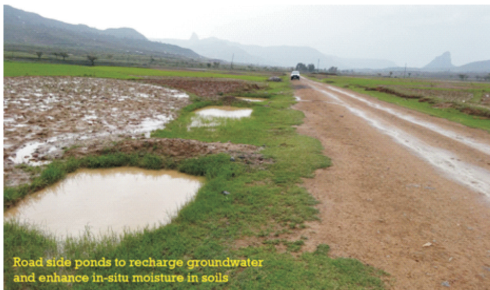
Plate 1: Road side ponds to recharge groundwater and enhance in situ moisture in soils
