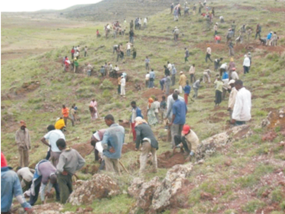
Plate 4: Community Mobilization to construct ridges, micro-pits, pits with manure and water dams
