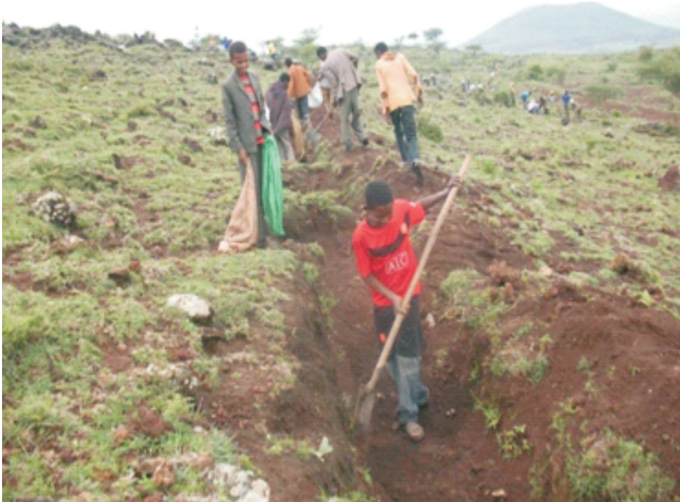
Plate 6: trenches to control run off water
